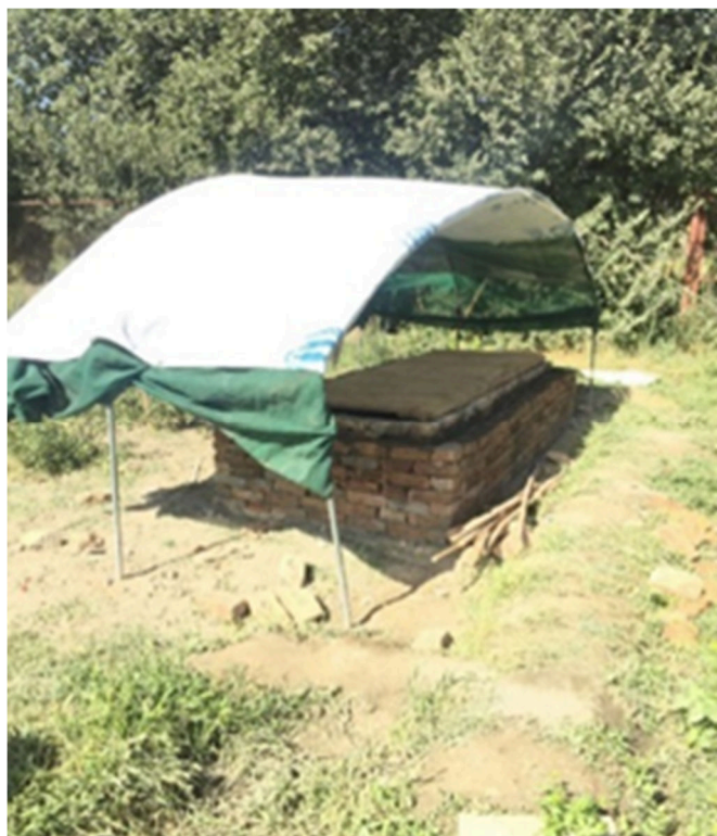
Figure 3. ZECC construction and related water tank completed.
