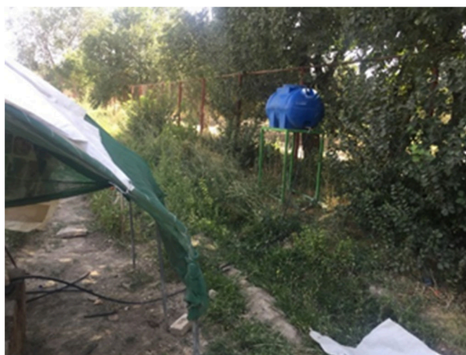
Figure 2. ZECC construction and related water tank.
